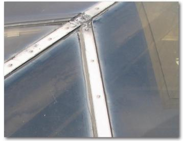
Recaulking over the years had not stopped the leaks and left a slightly messy appearance. Installation of the patented silicone gasket overlay system over the upper left portion of the skylight framework provided a clean appearance while eliminating potential for leaks.
