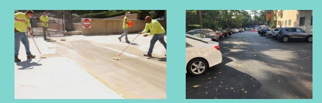
After the TREMProof<sup>®</sup> PUMA system was applied, asphalt was installed overtop and the lot was opened to traffic.
