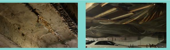
Water infiltration led to concrete deterioration and rusting metal, a big eye sore for occupants.
